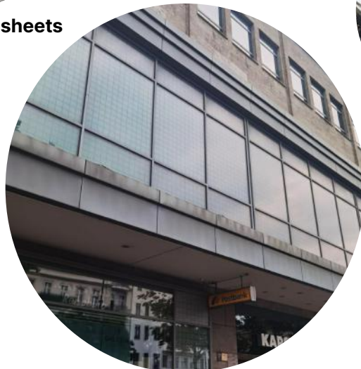
Post and beam facade
